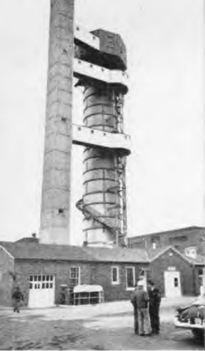
Training tank towers above base, contains 250,000 gallons of water.
